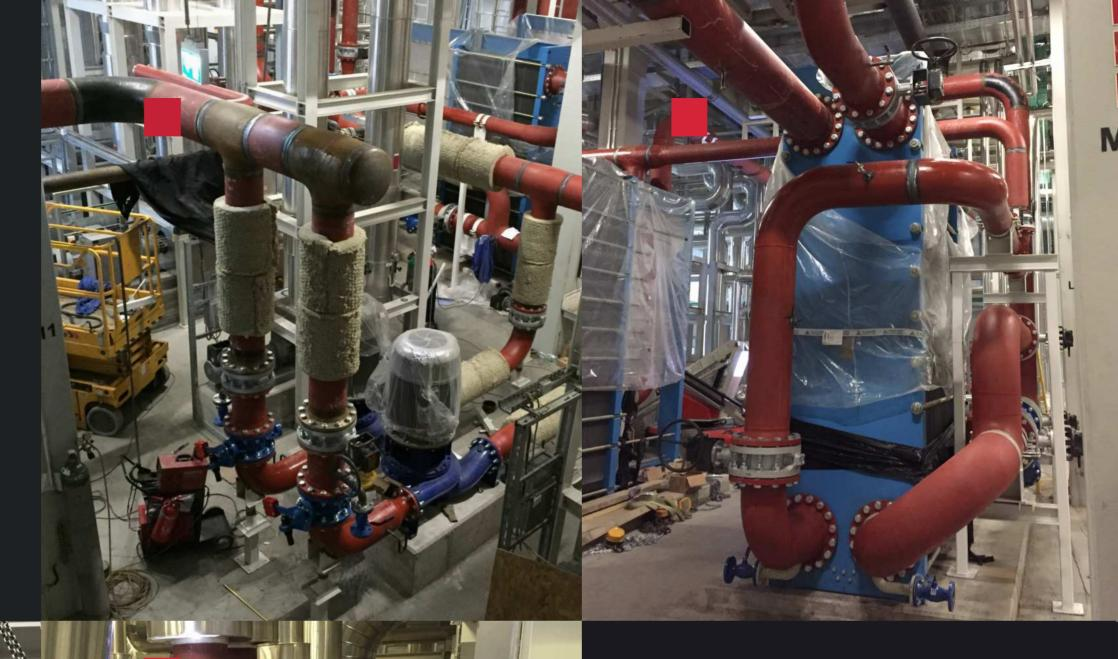
**CONSTRUCTION OF LIGHT WATER CONCRETE PLUMBING SYSTEMS** from acid-resistant pipe of material quality 1.4404, sizes DN100 - DN300
